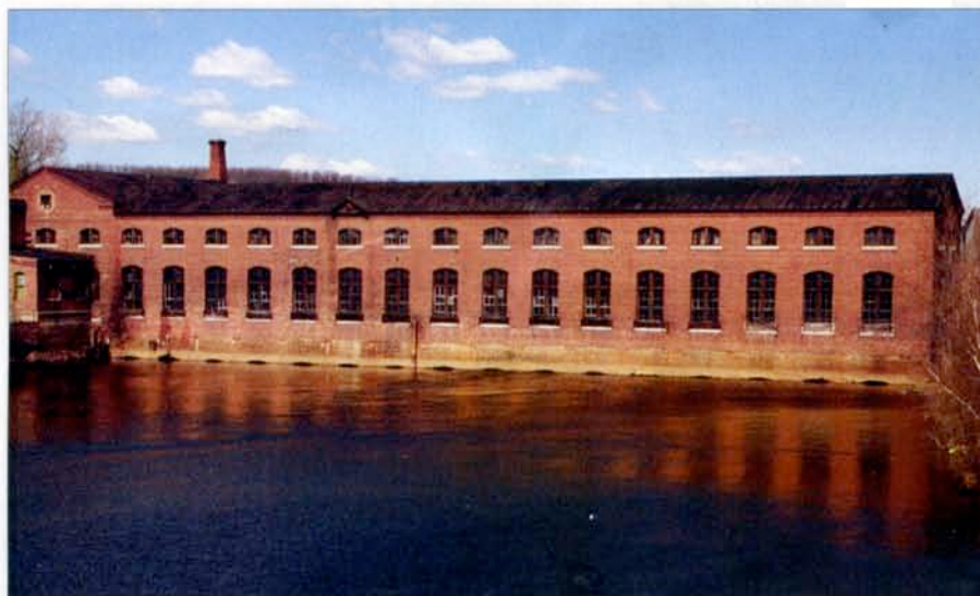
The generator hall straddles the Hudson River. The turbines sit beneath the building
