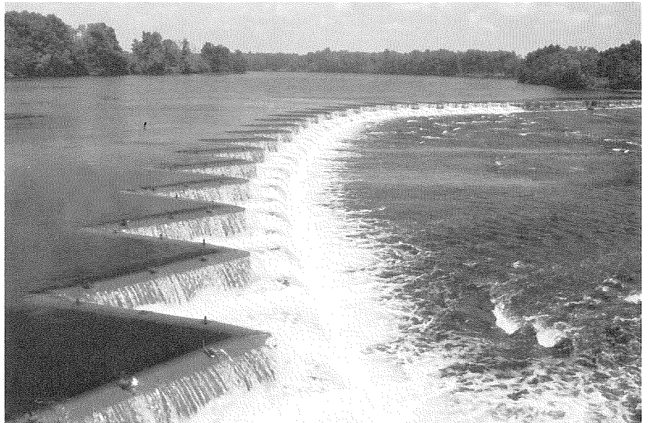
FIGURE 2: Precast labyrinth dam answered several hydraulic and scheduling problems.
